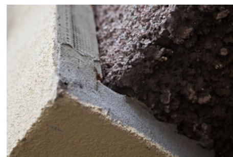
Close-up of external wall insulation.
