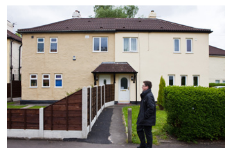
The house on the right has been refurbished by Northwards including external wall insulation.
