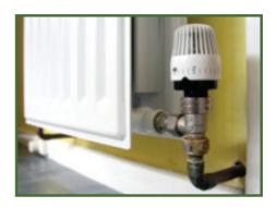
Turning these down can save money on your heating. This valve, fitted to your radiator, controls the temperature of the room where it is fitted. The higher the number the hotter the room. You can set the temperature of individual rooms with these controls. So if you're not using a room, turn the thermostat right down to save money.
